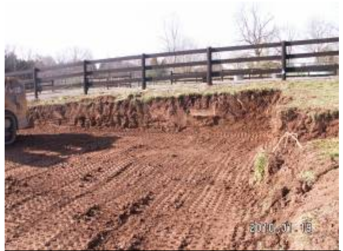
Grading the site for our "top-down" composter
