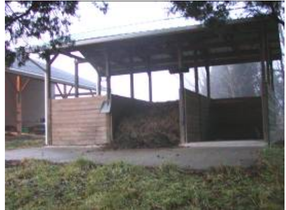
Standard government design w/manual aeration, full roof, and concrete pad
