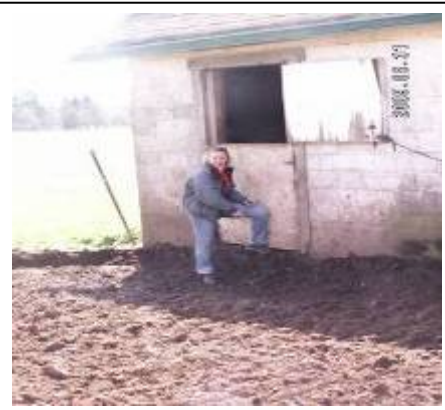
We removed more than a foot of organic muck and replaced it with bluestone gravel dust.
