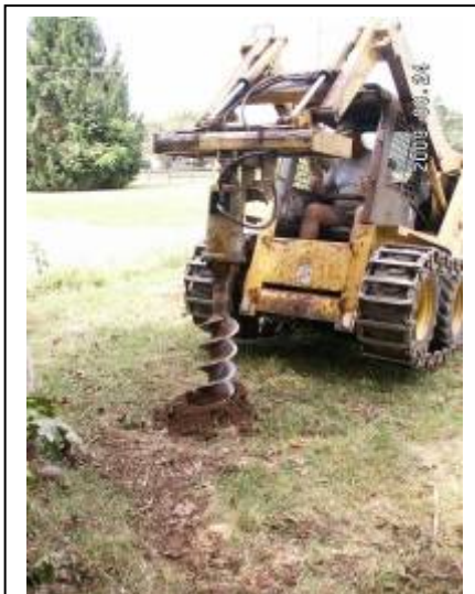
We dug the posts where necessary
