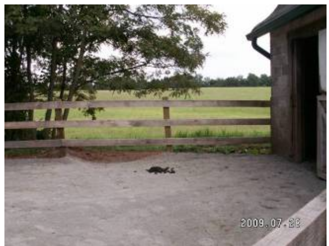
This is one of two swales installed to re-direct the rainwater.
