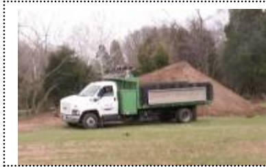
Trucking the topsoil away
