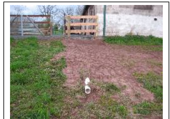
New gutters and downspouts redirect roof runoff to hayfield
