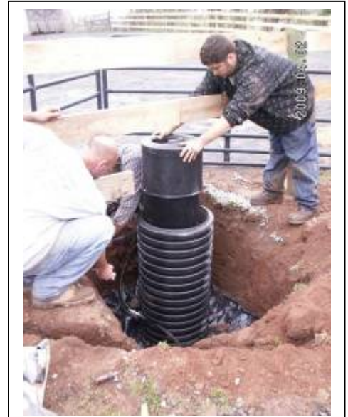
Site prep for our Bar-Bar-A water trough
