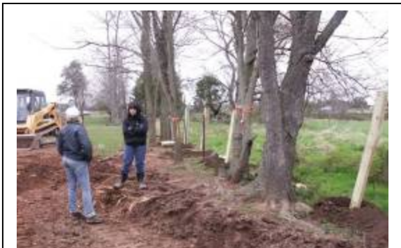
Some trees might not survive the excavation for the paddock
