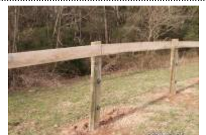
Streamside buffer fence right after fencing
