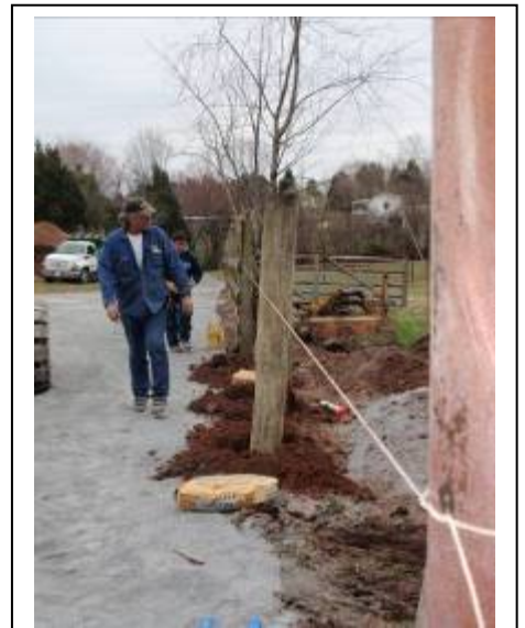
Board fencing installation around sacrifice area paddocks
