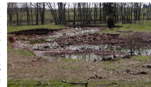
Erosion along a stream bank
