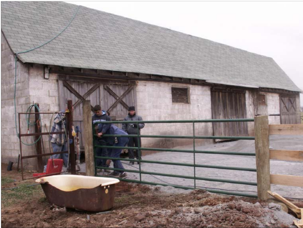
Installing 14' gate in back sacrifice area. Gate leads to driveway.
